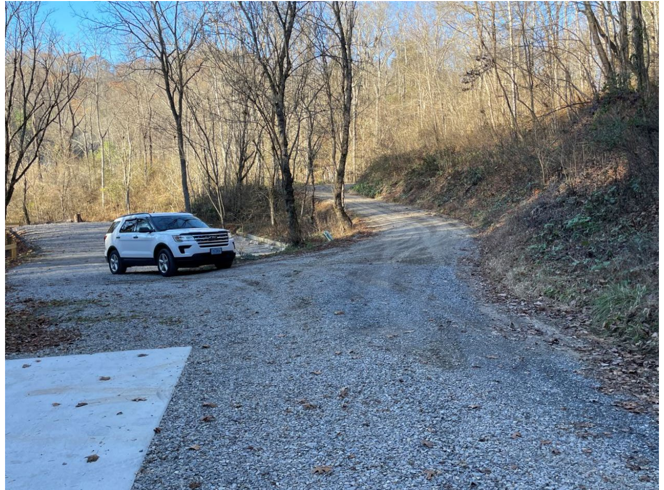
Viewpoint: Tank Hollow Road looking north
