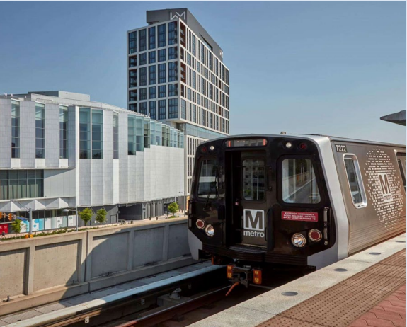
McLean Metro Rail Station, Fairfax County
