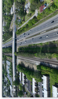
An existing section of Interstate 64 at Denbigh Boulevard where new eastbound on- and off-ramps will be constructed and the Denbigh Boulevard bridge will be widened as part of the Phase 2 project.
