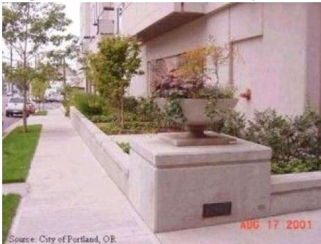
Figure P-FIL-05 B-1 Stormwater planters
