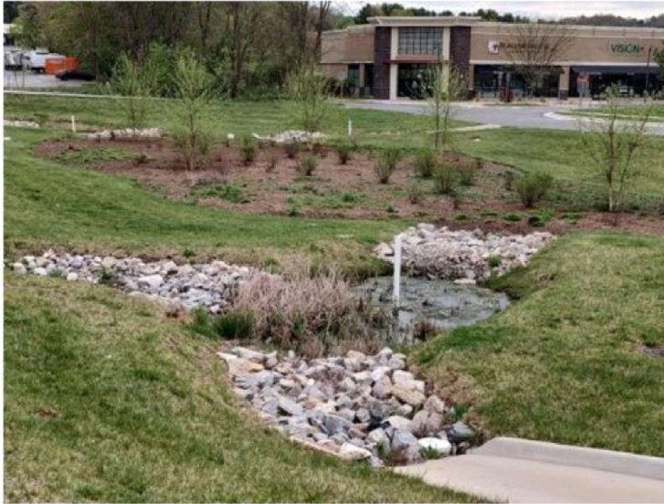
Figure P-FIL-05-3 Image of bioretention cell receiving stormwater runoff from multiple input points (3) in a mixed-use development in Blacksburg, VA
