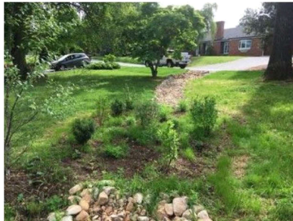
A residential bioretention used to manage upgradient street runoff that was formerly causing nuisance flooding downstream Photo Credit: Hirschman Water & Environment, LLC.
