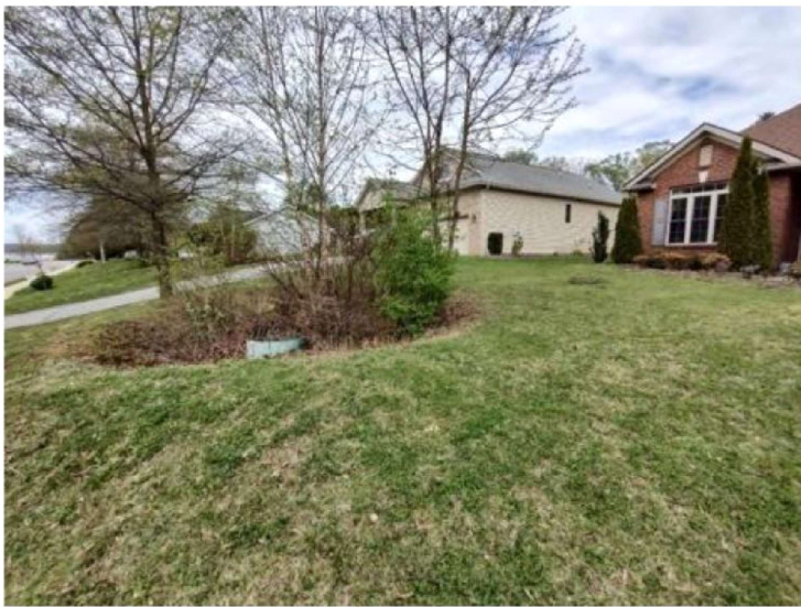
Figure P-FIL-05-4 Image of a micro-bioretention/rain garden cell receiving direct roof downspout input in Blacksburg Virginia
