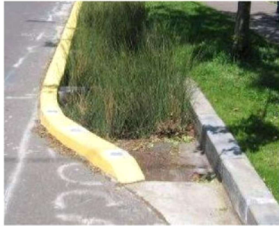
Figure P-FIL-05 B-3 Stormwater curb extensions
