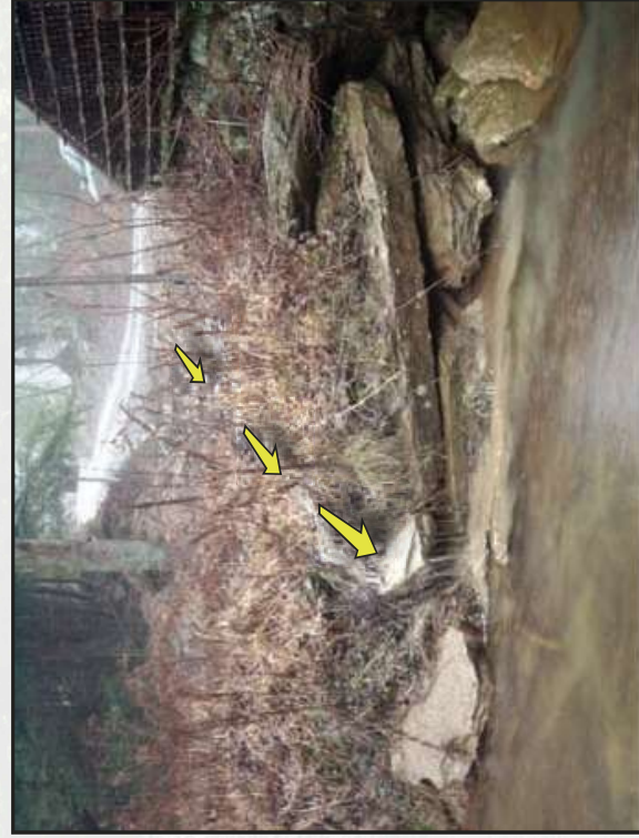
Figure 4.20—Traditional urban stormwater approaches collect and convey ditches directly to streams, as pictured above. Modern rural stormwater management should disconnect the road and stream by avoiding concentrated discharges to streams and encourage drainage dispersal.
