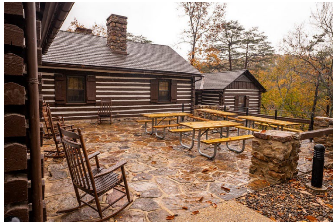
Figure 2: The newly renovated CCC-era lodge at Douthat State Park
