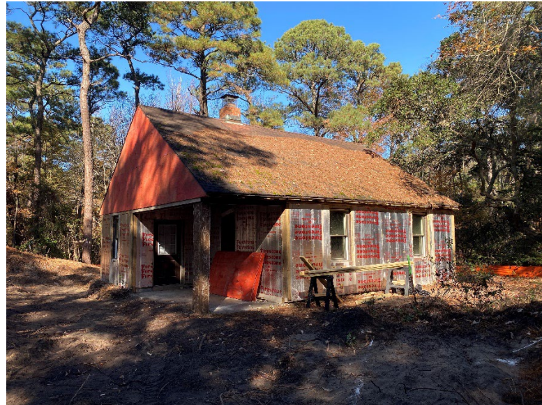
Figure 4: First Landing State Park :Cabin construction
